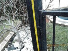
Are there any gaps in the barrier uprights on the inside greater than 10mm less than 100mm?
