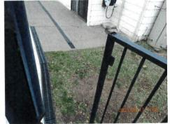
If a closed gate is lifted or pulled with a force of 250N, do any of the following occur. Release the latching device?. Unhinge the gate? Or Increase gap below barrier by more than 100 mm?
